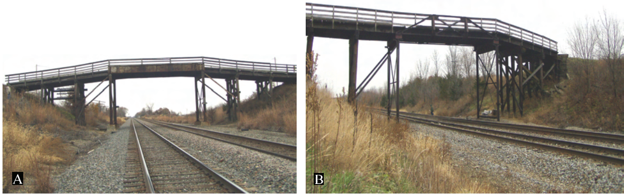
Figure 92. Late 19 th to early 20 th century combination wooden and steel trestle railroad overpasses along old U.S. 34 near Lockridge. A. Bridge that was part of the Blue Grass Road by 1913. B. Former township road and livestock overpass now closed to traffic. Note jog in middle. 2003 survey photos.
