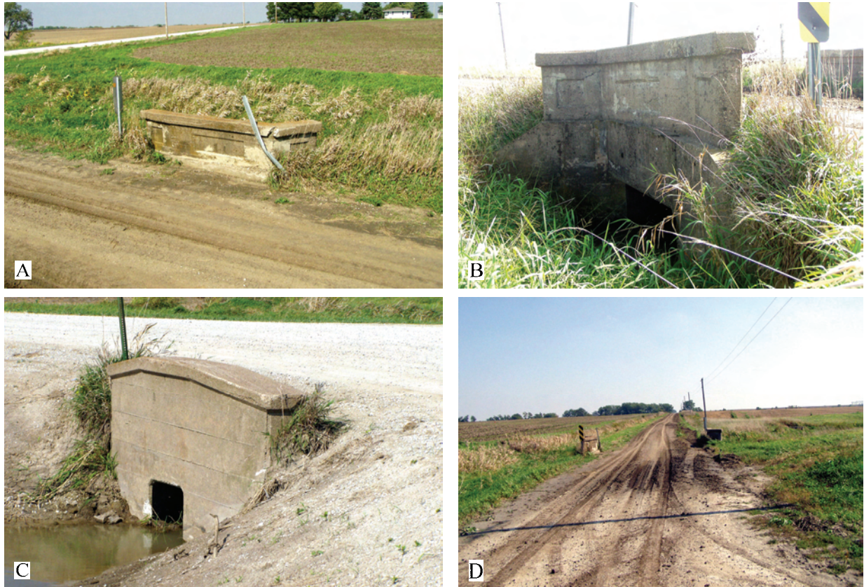
Figure 86. A. The dated 1916 Blue Grass Road signature culvert using standard state design, New London vicinity, Henry County. B. Side view of same. C. County-built parapet top culvert (1929) on Blue Grass north of New London, Henry County. D. Viewshed photo showing segment unimproved since 1916. All located at corner of Oasis Avenue and 240 th Street northwest of New London. 2005 photos.
