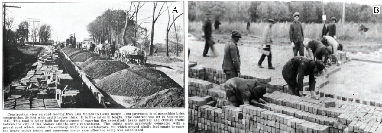
Figure 22. A. Material set up on the Des Moines to Camp Dodge Road in 1917 (ISHC 1917d:inside front cover). B. Workers laying the Des Moines to Camp Dodge Road (1917–1918) (Thompson 1989:146).
