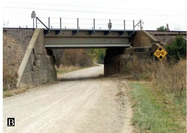
Figure 89. A. View of the Rome vicinity gravel segment of 1912 Blue Grass Road. B. Associated concrete railroad underpass that retains the painted Blue Grass Route sign illustrated in Figure 67. Like most such structures the top has been replaced or rebuilt. 2003 survey photos.
