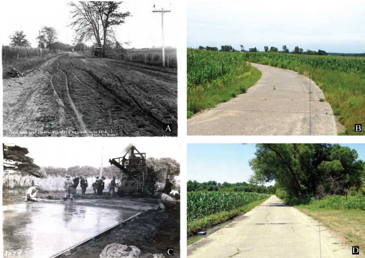
Figure. 71. A. The Fredonia to Columbus Junction sand road prior to experimental 1916 concrete paving. Photo by Baker (ISHC 1916c). B. Current view-shed photo of west end of pavement (2003 survey photo). Note B is the same view as A. C. Paving in progress using convict labor (1916) (ISHC 1916c, Photo #3079). D. Current view-shed of west end pavement (2003 survey photo).
