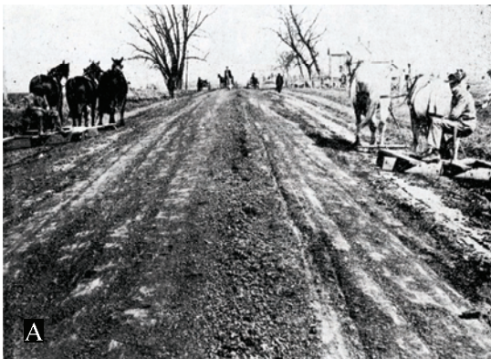
Figure 24. A. After Dragging in Jackson Township, Hardin County (Road-Maker 1916c:27) Note use of four drags. B. Iowa road crew dragging road with a traction engine in 1915 (Road-Maker 1915b:6).
