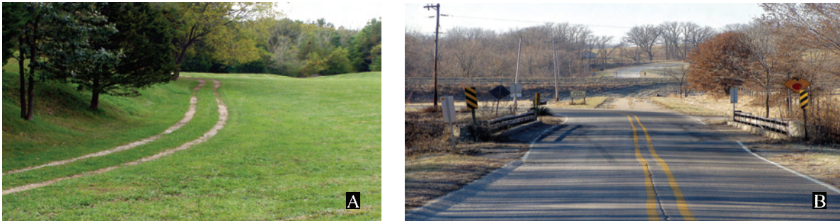
Figure 99. A. View of route of 1900 to 1916 Blue Grass Road skirting Albia cemetery. B. Cut-off concrete highway segment west of Albia, Jefferson County at intersection of old U.S. 34 and current U.S. 34. Note curb, new turn before 100 ft cut-off segment, current U.S. 34 grade, then resumption of old U.S. 34.
