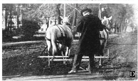
Fig. 23, A "Good Roads Special" Demonstration Bloomfield, Iowa, Nov. 1, 1905. Mr. D. Ward King and the "Split Log Drag."
