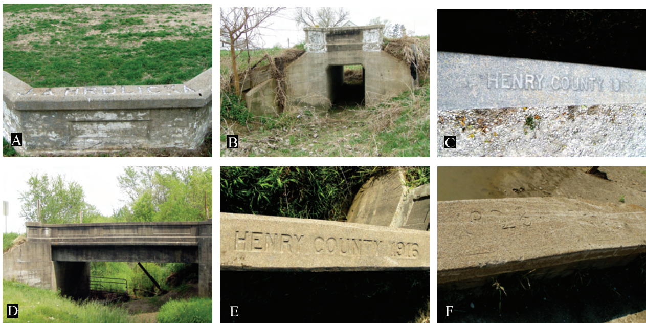
Figure 56. A. “HRDLICKA” impressed signature livestock culvert on Red Ball/old U.S. 218, North Liberty vicinity, Johnson County. B. View of west side (A–B 2003 survey photos). C. “HENRY COUNTY 1917” culvert on Blue Grass Road. D. View of west side. Note use of standard 1913 ISHC design. E. “HENRY COUNTRY 1916” Blue Grass Road siderail culvert using same template, New London vicinity, Henry County. Note edge chamfer. F. Henry County signature culvert incised “1928-Henry Co.-L.E.,” New London vicinity (C–F 2005 photos). Note A–E are derived from the ISHC 1913 stand culvert plan.
