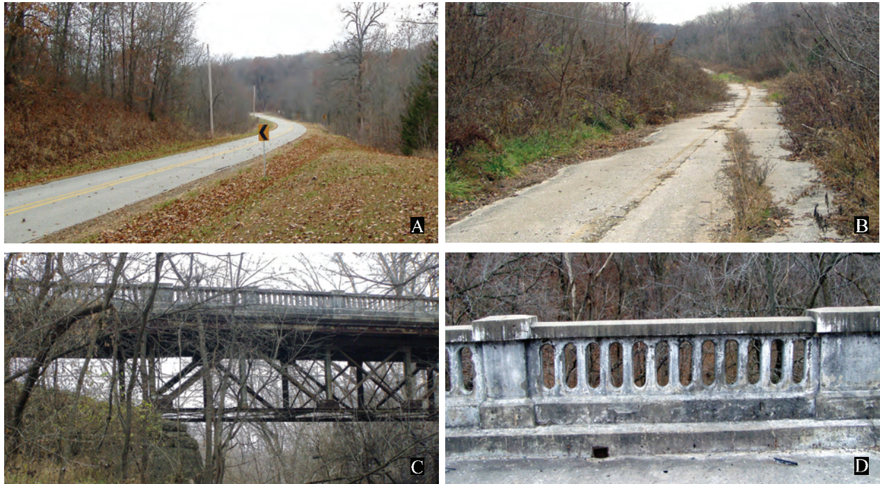
Figure 95. A. View of in-use, asphalt surfaced Segment 1 atop old railroad grade looking southwest. B. View of abandoned Segment 2 looking southwest. C. View of abandoned deck-truss bridge on Segment 2 with 1869 stone footings. D. Detail of bridge handrail. 2003 survey photos, Ottumwa, Wapello County.
