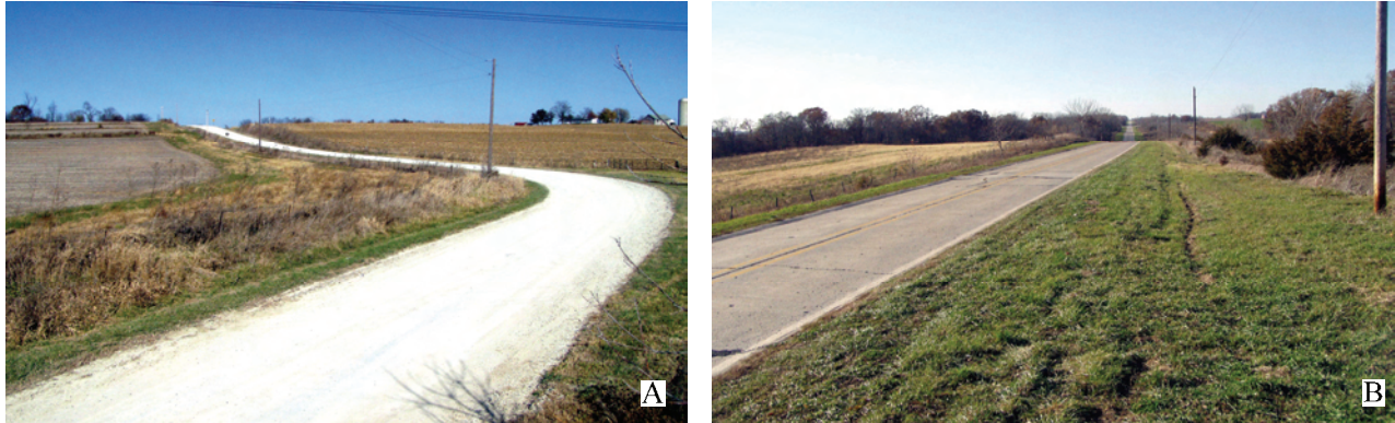
Figure 12. A. Decommissioned in-use 1910s–1920s segment of Blue Grass brought to grade and graveled, Lockridge vicinity, Jefferson County. B. Cut-off and in use 1920s–1930s era concrete surfaced segment of U.S. 34, Lockridge vicinity, Jefferson County. 2003 survey photos.
