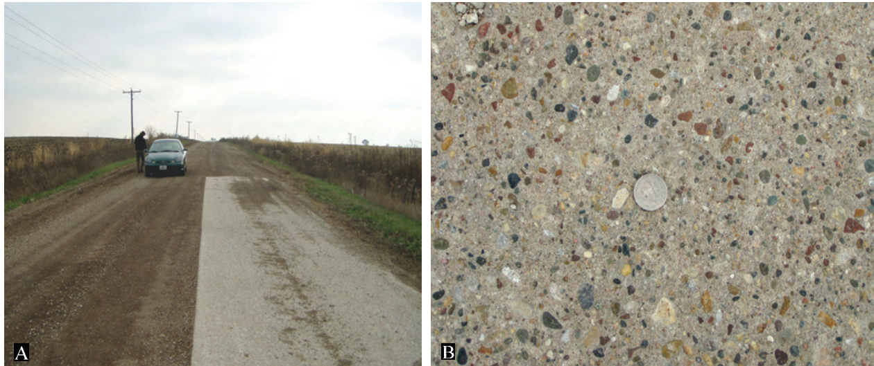
Figure 85. A. View of the end of the Half-Slab near Bonaparte, Van Buren County. B. Detail of ca. 1948 pavement of same with sorted river gravel in poor quality aggregate. 2003 survey photos.
