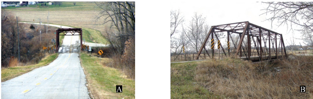
Figure 98. A. View in 2003 of the ca. 1928 Avery Creek bridge (nonextant 2005) in Wapello County. Note asphalt over-paving between original concrete curbs. B. View of same looking east. 2003 survey photos.
