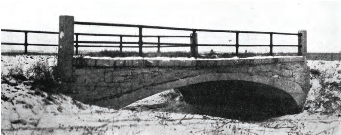
Figure 1. The 1893 Lyon County bridge. The first reinforced concrete arch bridge in the country (ISHC 1915a:55).
