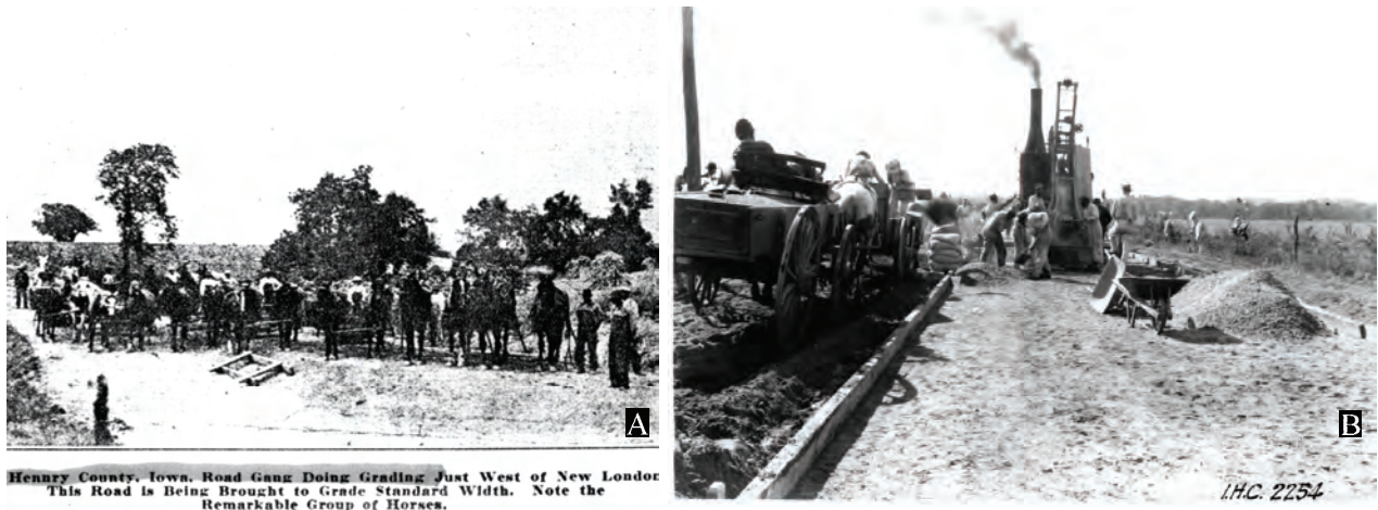
Figure 25. A. Henry County road gang working on the Blue Grass Road near New London ca. 1914 (Road-Maker 1914e:6). B. Fredonia to Columbus Junction Road convict paving gangs in 1914 (Iowa DOT Library–Paving Folder, Photo #2254).
