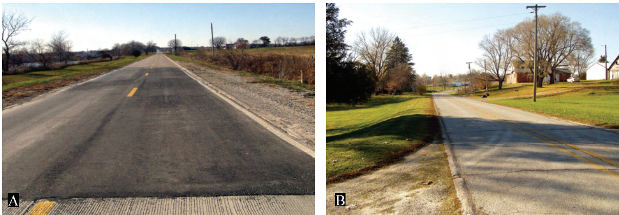
Figure 14. A. View of in-place cut-off segment on old U.S. 34, Lockridge vicinity, Jefferson County. B. View of integral lip-curbed segment on old U.S. 34, Rome, Henry County. 2003 survey photos.
