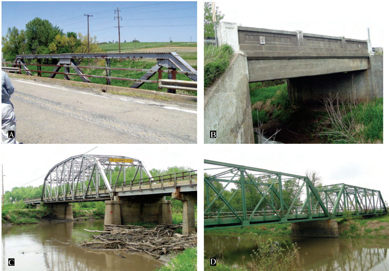
Figure 108. A. The Davis Creek pony truss bridge (nonextant 2005) on old U.S. 218 south of Iowa City. B. Art Moderne style bridge over secondary drainage into Old Man's Creek (2003 survey photo). C. Old Man's Creek bridge (nonextant 2005). D. English River bridge (nonextant 2005). 2003 survey photos.
