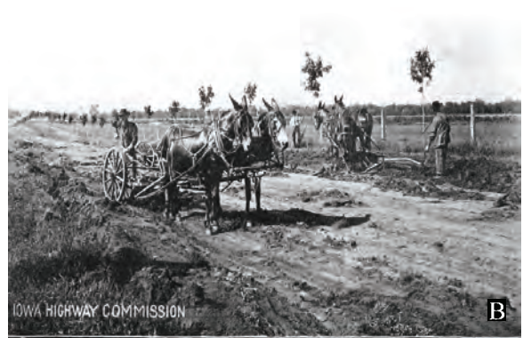
Fig. 21 The Making of an Earth Road. Road School—Ames, June 15th to 17th. The work was completed with a reversible grader. Outfit owned and work done by C. D. Goetze, Coos Rapids, Iowa.
