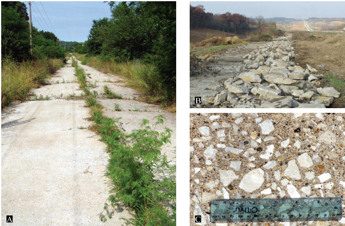
Figure 104. A. View of original cut-off 1928 segment at the Skunk River south of Mount Pleasant, Henry County. B. View of same old segment being broken for rip-rap. C. Detail of 1928 aggregate showing use of dolomite and finely sorted natural and crushed river gravels. 2003 survey photos with 6" ruler.
