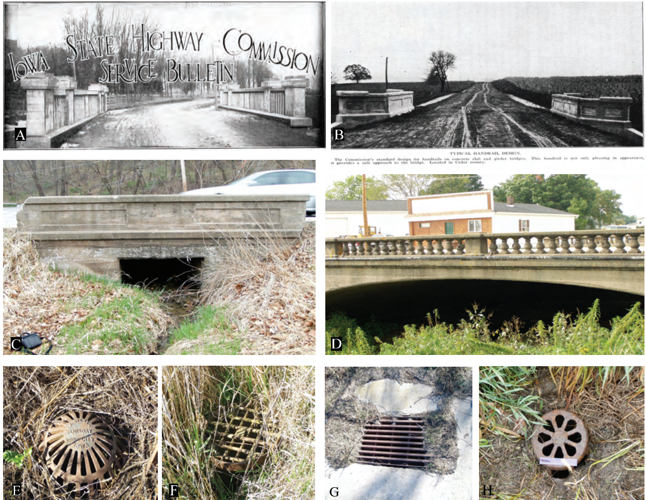
Figure 58. A. Cover photo of handrail culvert from ISHC Service Bulletins (ISHC 1926a:cover). B. ISHC Standard Design for handrail on concrete and girder bridges (Cedar County) (ISHC 1915c:53). C. Siderail of ca. 1911 culvert from the Red Ball Route, Dubuque Street, Iowa City (2003 survey photo). D. Balustraded handrail on Stark-built arch bridge in West Union, Fayette County (2003 survey photo). E. Beehive shaped drain inlet cover made in Iowa City, old U.S. 34, Henry County. F. Hand welded inlet cover made of round rebar on old U.S. 34, Henry County. G. Welded flat grate drain inlet, old U.S. 34, Jefferson County. H. Cast iron inlet cover from old U.S. 34 near Ottumwa, Wapello County (6" ruler).
