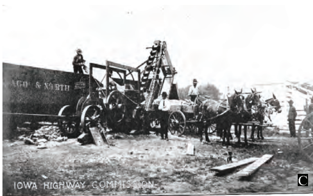
Fig. 22 Stone crusher at work during road school.
