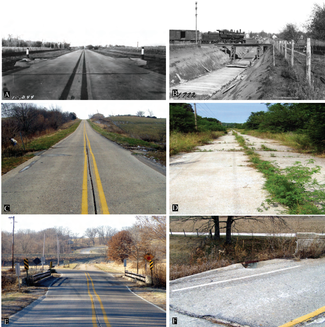
Figure 61. A. Circa 1926 integral lip-curbed rural highway (Iowa DOT Library–Paving Folder, Photo #13,244). B. A 1920s below grade curbed crossing and new overpass. Note pavement’s covering of earth and wet burlap (Iowa DOT Library–Paving Folder, Photo #11,722). C. Integral lip-curbed rural highway segment with integral drains along old U.S. 34 near Albia (ca. 1928). D. A ca. 1928 integral lip-curbed rural highway segment along old U.S. 218 (Red Ball) near Mount Pleasant (nonextant 2003). E. Current intersection of integral lip-curbed segment of old U.S. 34 cut by current U.S. 34 with replacement paving, approach, and bridge. F. Old U.S. 218 (South Curtis Bridge Road, Johnson County) exhibiting integral lip-curb with integral drain inlet just past culvert. Figures C–F are 2003 survey photos.
