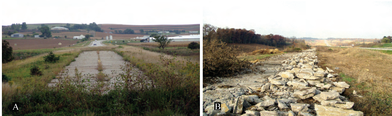
Figure 15. A. Cut-off segment of old U.S. 92, Mapleton, Monona County. B View of old U.S. 218 (ca. 1930) broken-up for reuse as bridge rip-rap, Mount Pleasant vicinity, Henry County. 2003 survey photos.
