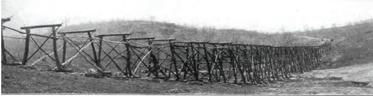
Wooden trestle made of chopped timber
