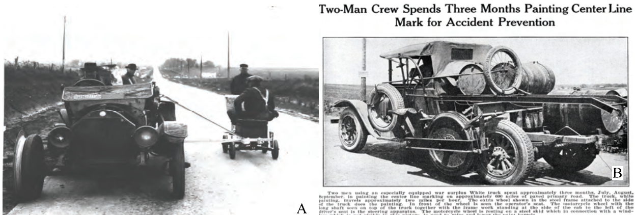
Figure 68. A. Center line painting in 1923. Reverse of photo notes car as a Maytag (Iowa DOT Library–Photos). B. Center line painting truck in 1926 (ISHC 1926f:5). Note motorcycle wheel in back.
