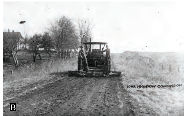
Figure 24. A. After Dragging in Jackson Township, Hardin County (Road-Maker 1916c:27) Note use of four drags. B. Iowa road crew dragging road with a traction engine in 1915 (Road-Maker 1915b:6).
