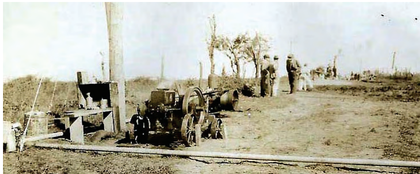
Figure 29. Convicts and water pump on the Fredonia to Columbus Junction section of the Blue Grass Road ca. 1914 (ISHC 1914c).
