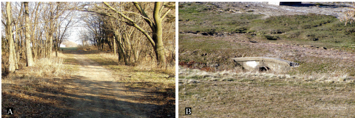
Figure 16. A. Segment of the Airline Highway (1900s–1920s) now a field access (later Iowa 8) east of Albia cut off in the 1930s. B. Contributing cut-off segment of a pre-Civil War road used as part of the Airline Highway (ca. 1916–1925) with early parapet culvert visible from old U.S. 34. 2003 survey photos.
