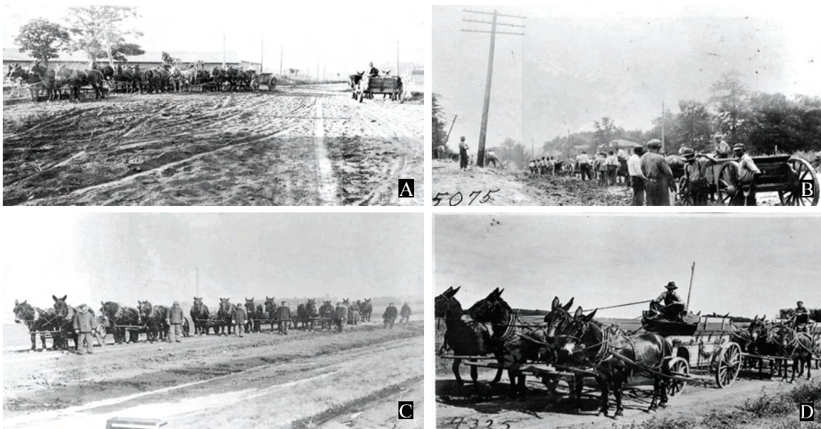
Figure 37. A to D. Washington County road crews at work along or near the Red Ball Route using horse-drawn elevating graders and other equipment (Photos B #5075 and D #4325, Iowa DOT Library).
