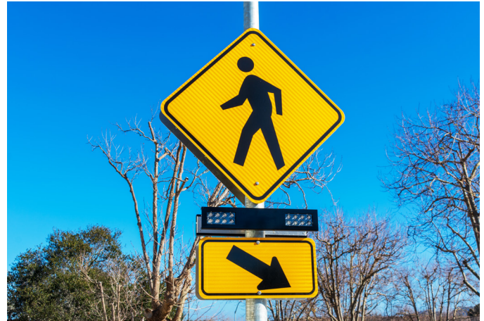
Figure 2.12: Rectangular rapid flashing beacon
