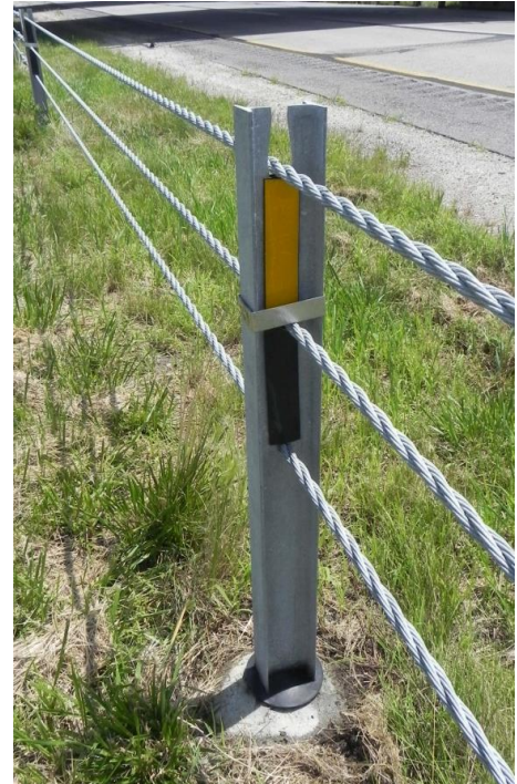
High tension cable guardrail example
